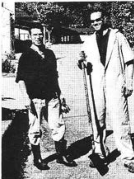
Paradise Park crew members Philippe Ezanno (left) and Jeremy Hewitt can be seen doing all kinds of repair work around the park. Here, they are filling in asphalt for some road repair. Thanks, guys, for the smiles!
